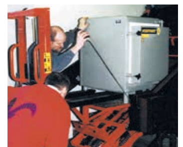
Professional installers moving a chamber kiln into a basement studio.
